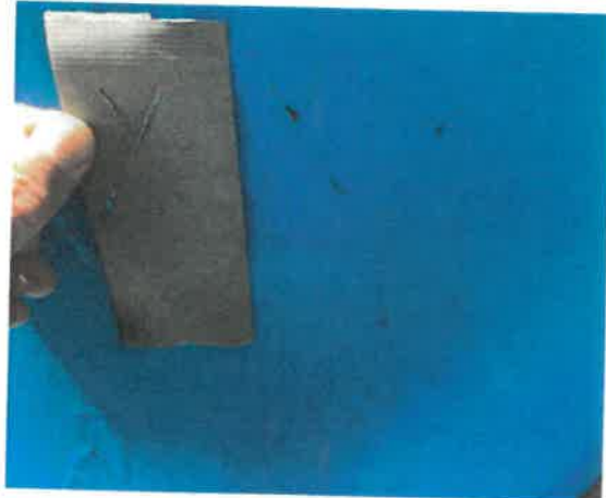
PHOTO #2: Adhesion test south tower leg.
