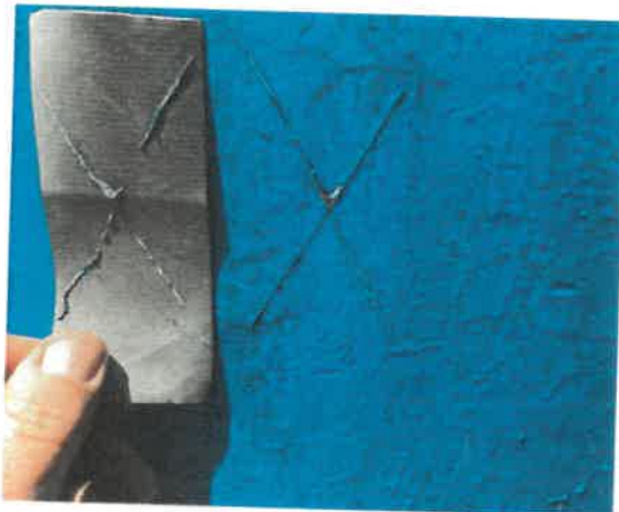
PHOTO #5: Adhesion test south side of riser.
