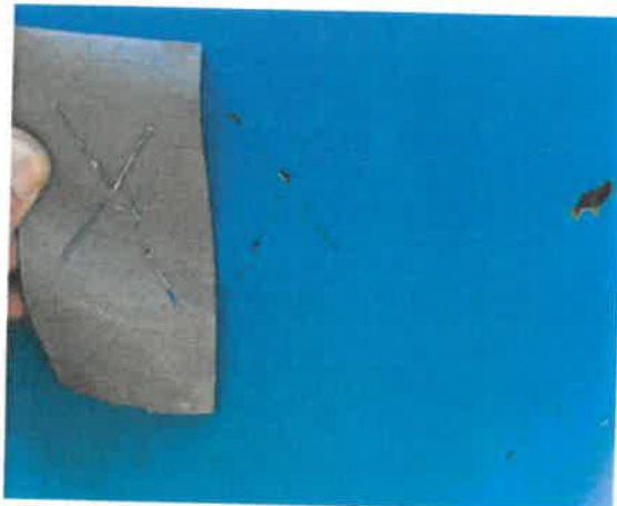
PHOTO #3: Adhesion test north tower leg.
