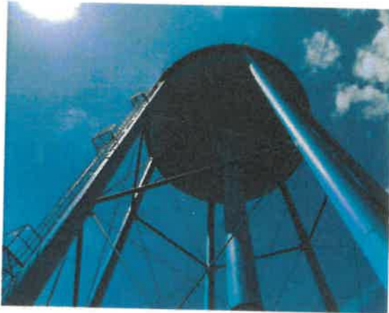
PHOTO #1: 500,000 gallon toroellipse (North) tower.
